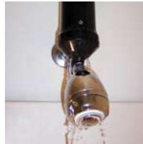
**Note:** In case severe sediment levels or neglect has caused slow water flow, a power backwash may be necessary. With water running, simply rotate the filter cartridge back and forth between backwash and service settings quickly and repeatedly. Do this until water flow is restored and then for at least one minute longer.
